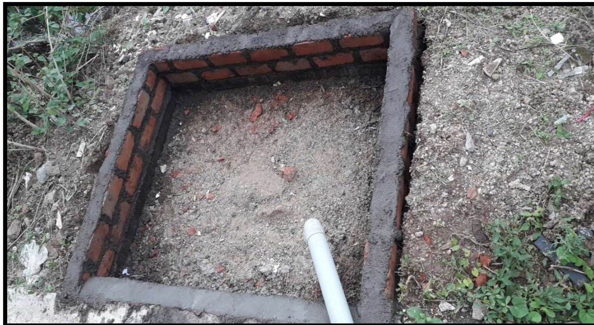
Soak pit for Chemistry laboratory hazardous waste water
